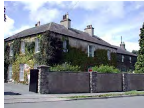
Beechgrove House, Dublin Street
