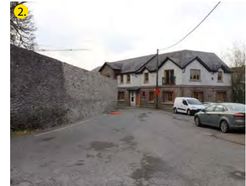
Fire Castle Gate Location
