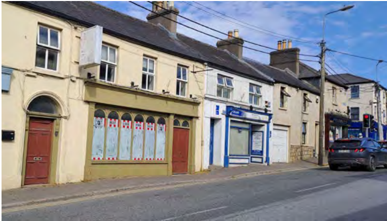
Vacant units on Bride Street
