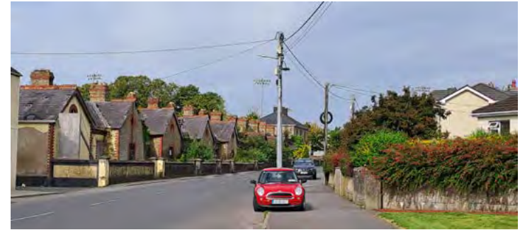
Existing Photos highlighting recent renovations and remaining dereliction on Shraud Street
