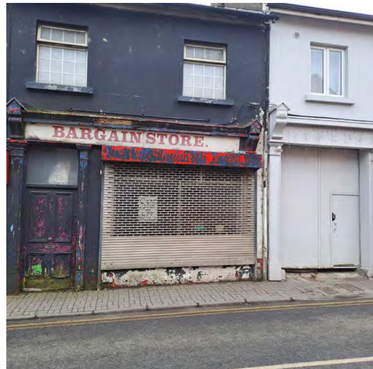
Vacant units on Bride Street
